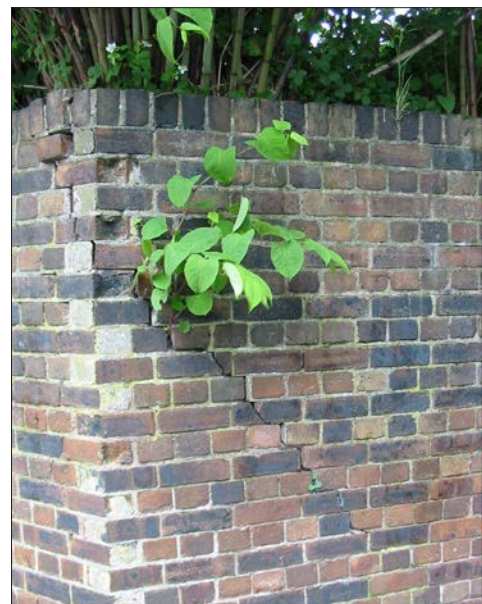
Figure 2-12. Knotweeds cause considerable damage to infrastructure (Credit: © Japanese Knotweed Solutions Ltd, www.jksl.com)
